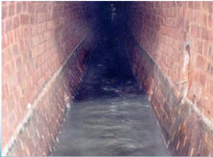
Free flowing egg shaped brick sewer
